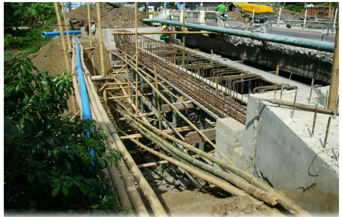
Relocation of 10 " Distribution Line along Box Culvert Crossing Under DPWH road widening project at Sibaguan- Balijuagan, Roxas City.
