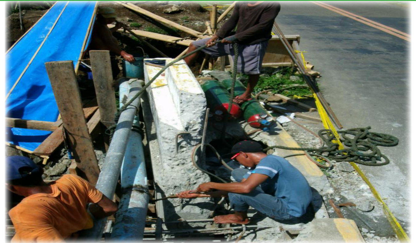
Relocation of 6 " Distribution Line along Bridge Crossing Under DPWH road widening project At Tadiao bridge, Panay. Capiz.
